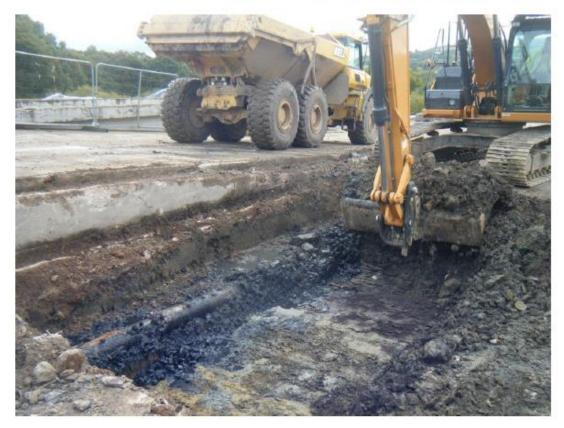
Diggers were able to chase out the contamination and impacted soils were sent off site for disposal.
