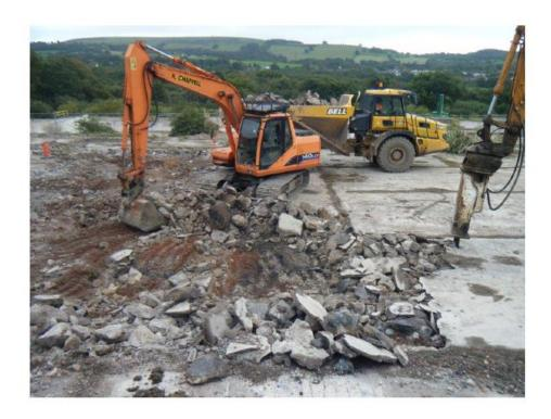
Areas of gross contamination were clearly visible and enabled these to be quickly identified and removed.
